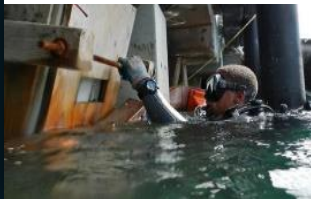
Dive Inspection Support
