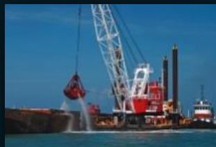
Dredging & Rock Dumping
