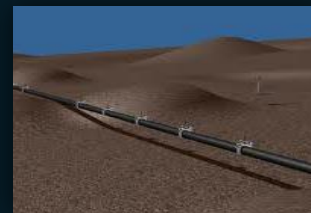
Pipeline Survey & Leak ID
