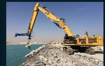
Breakwater Construction
