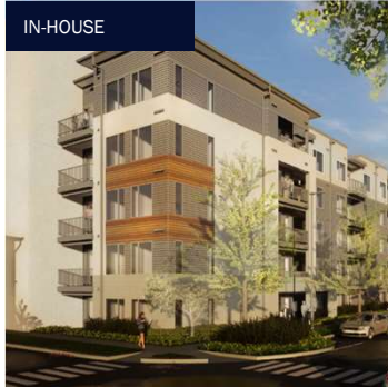
MAA Milepost 35 II | NOW LEASING Denver, CO
