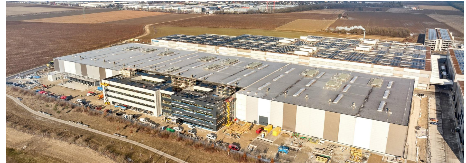
VGP Park München – Building D, Germany
