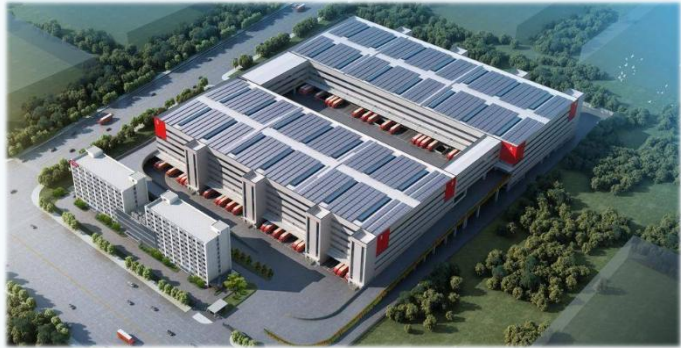
Yiwu Sorting Center under construction
