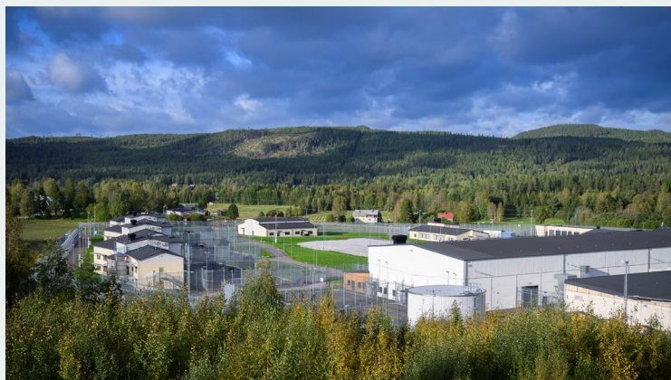
Prison, Ånge Estimated completion, Q4 2027
